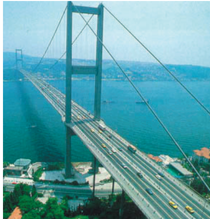
Figure B1: A suspension bridge
